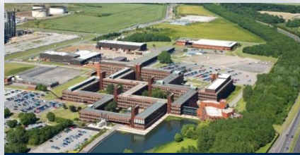
National Industrial Biotechnology Facility
