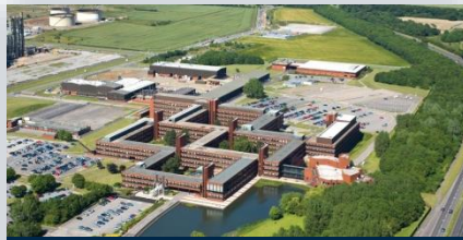
National Industrial Biotechnology Facility
