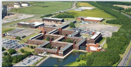
National Industrial Biotechnology Facility
